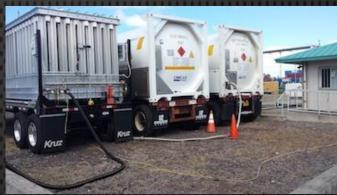
**Natural draft:** relies on wind and natural convective currents to move air over the units. As warm air comes into contact with the AAV cells, the air cools and becomes dense, causing it to flow downwards to the bottom of the cells. This causes the warm ambient air from the surroundings to be drawn through the top of the cells
